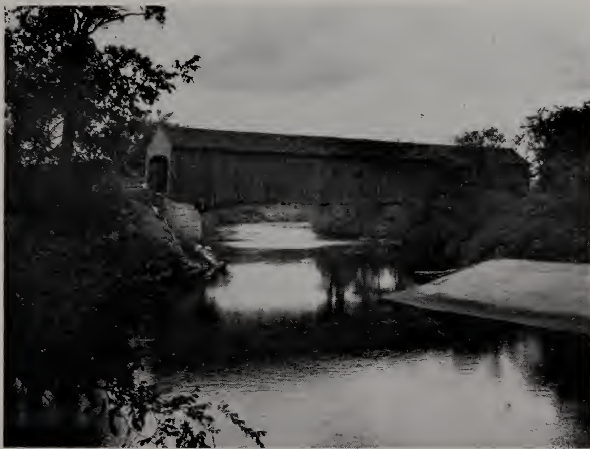
The lattice bridge of 1874 over the Baker River in the Village.
